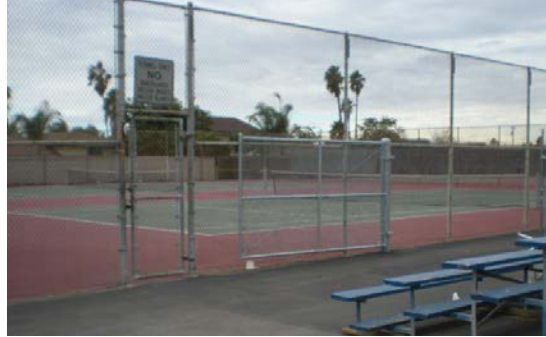
Need to refurbish tennis courts.
