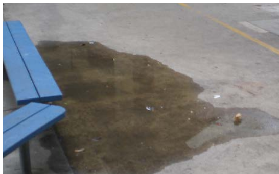
Ponding/drainage issues need to be addressed.
